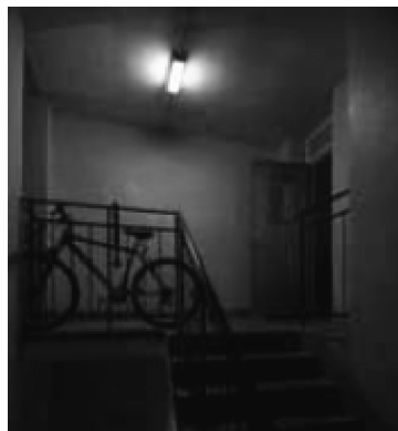
photo of stairwell with fluorescent fitting
